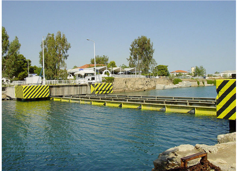
Image of submersible bridge over the Corinth Canal in Greece taken by Aspasia Coumiotis.
